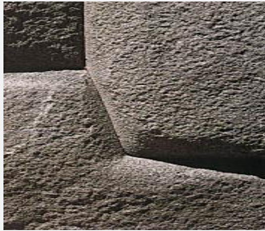
An Inca wall of carefully cut masonry that formed part of the palace of Inca Roca in Cuzco.
